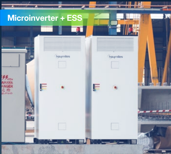
Location: Malaysia Capacity: 625 kW / 1,305 kWh Product: HoyUltra series Scenario: Concrete production facility Highlights: Hoymiles microinverter, lower energy cost
