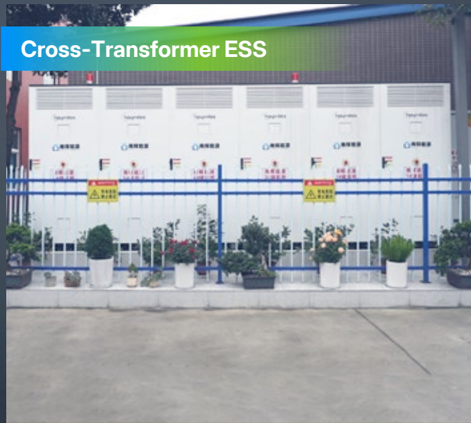
Location: Chengdu, Sichuan Capacity: 750 kW / 1,566 kWh Product: HoyUltra series Scenario: Factory Highlights: Peak-valley arbitrage, improved renewable consumption
